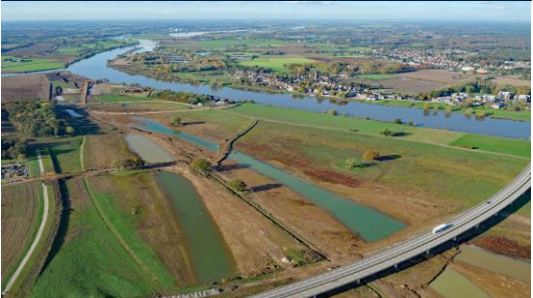
Levee reinforcement project won Dutch Water Innovation Award
