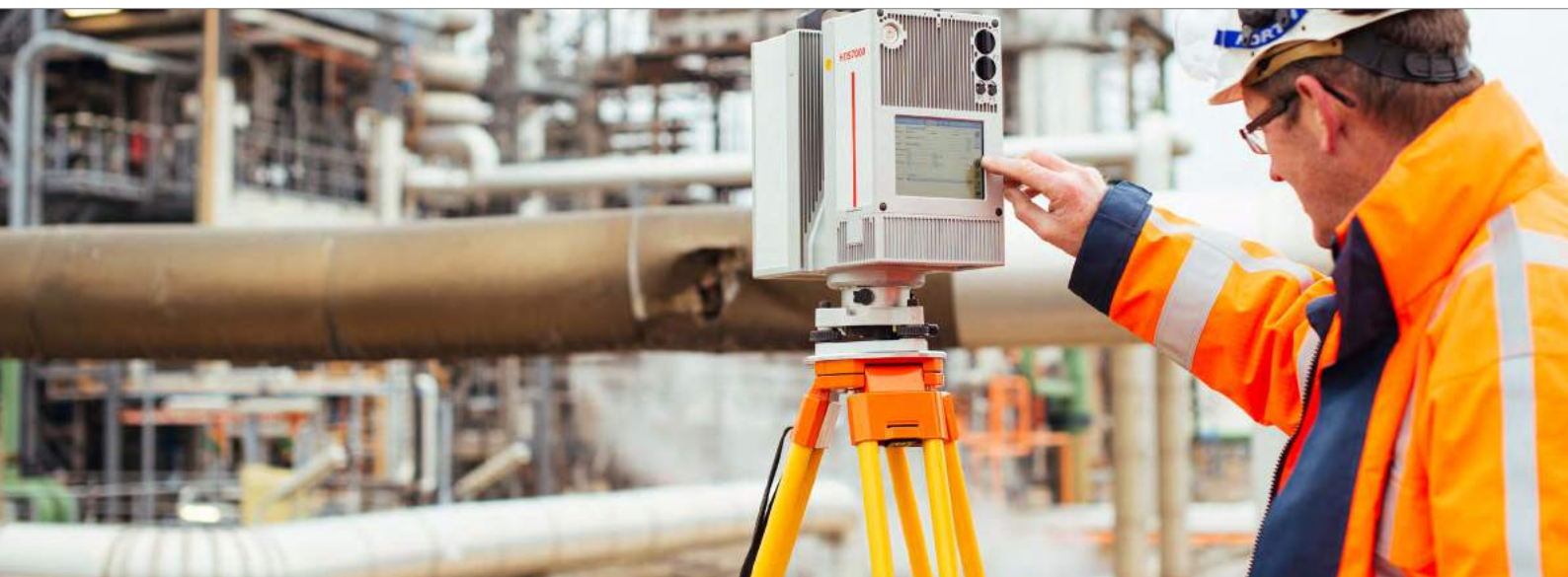
3D laser scanning of industrial facilities, Moerdijk, the Netherlands.
